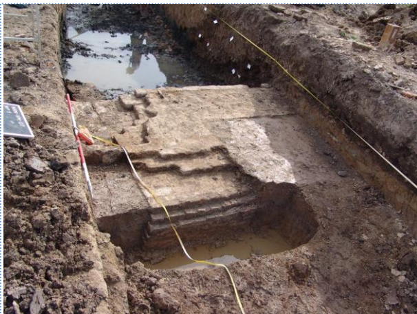
Fig. excavations at the castle
